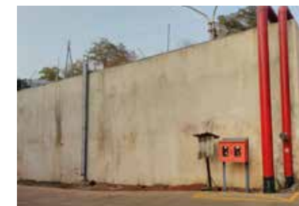
Dedicated water storage tank for fire fighting
