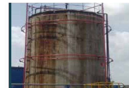
Sprinkler provision for methanol storage tank safety
